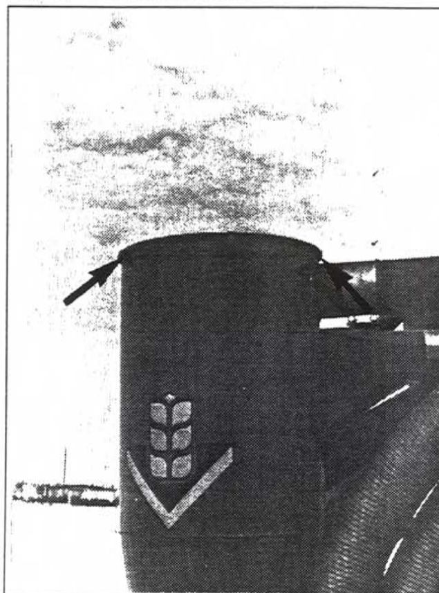
Fig. 42 SCREEN (under lid at top of BPS)
